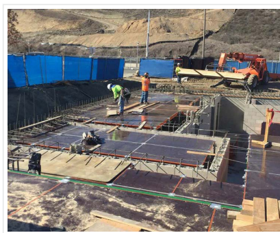
Green Formwork System
