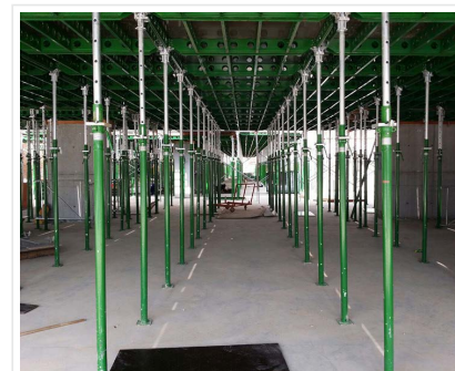
Green Formwork System
