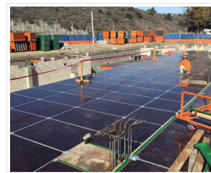
Green Formwork System
