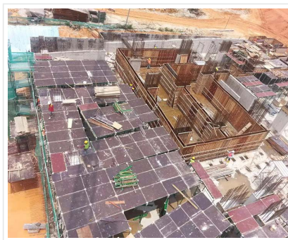
Green Formwork System
