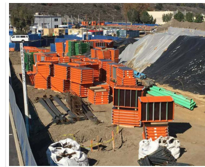
Green Formwork System
