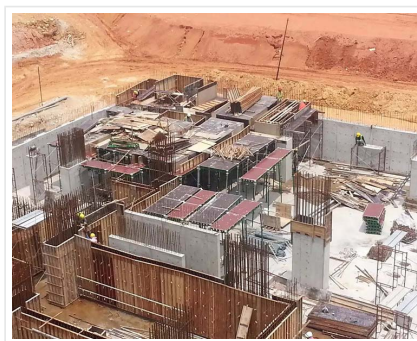
Green Formwork System
