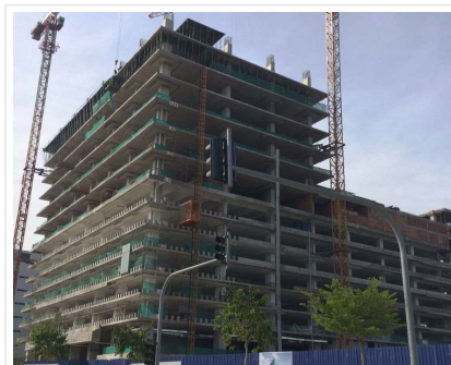
Green Formwork System
